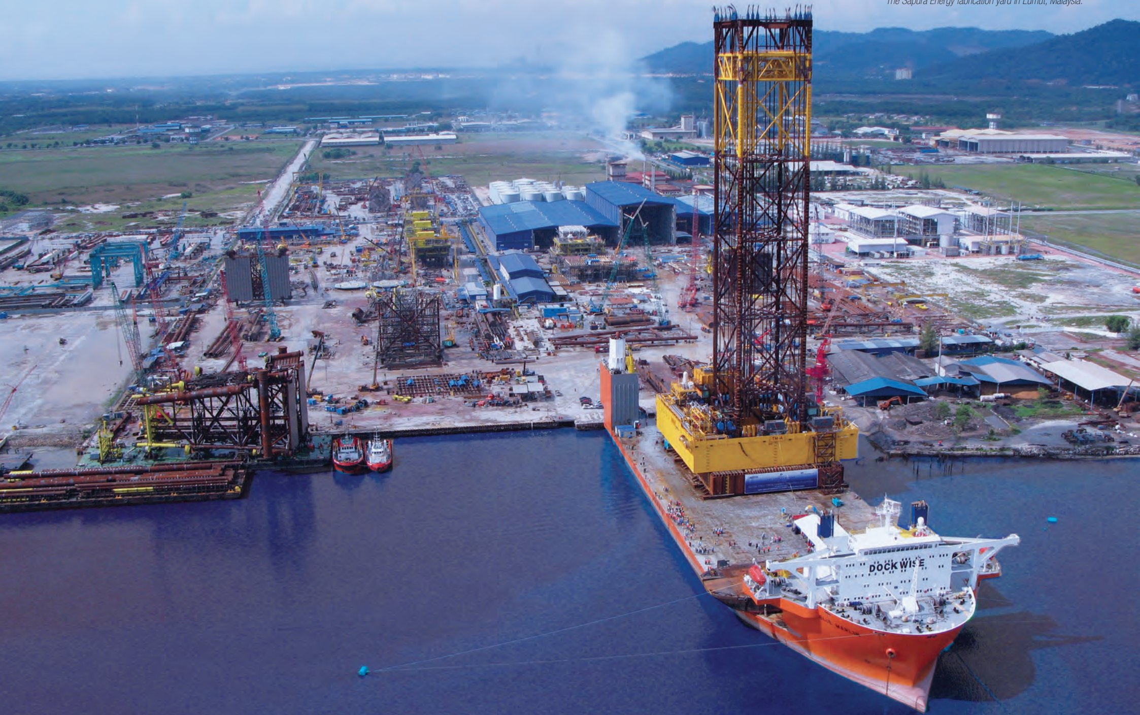
The Sapura Energy fabrication yard in Lumut, Malaysia.
